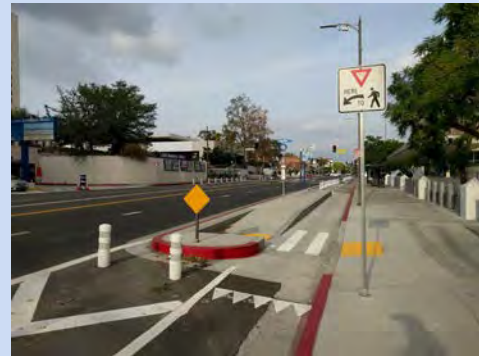
"Floating" Bus Stop and Protected Cycle Track (Los Angeles, CA)
