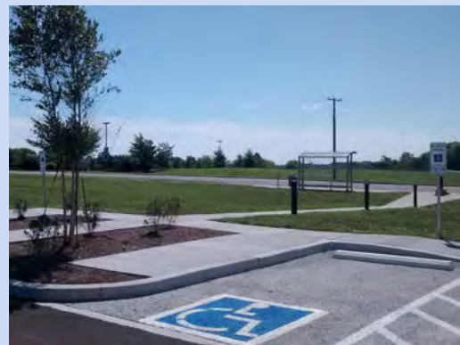
Accessible Features at Park-and-Ride Lot (Gallatin, TN)
